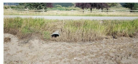
#49. VIEW OF EAST CULVERT
