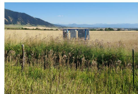
#44. VIEW OF NORTH ELECTRICAL, DITCH & FENCE
