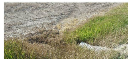
#50. VIEW OF EAST CULVERT
