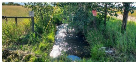
#48. VIEW OF NE CREEK, CULVERT, GATE AND FENCES
