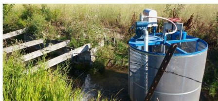
#45. VIEW OF NE HEADGATE
