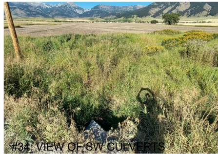
#34. VIEW OF SW CULVERTS
