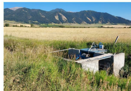
#39. VIEW OF NORTH HEADGATE
