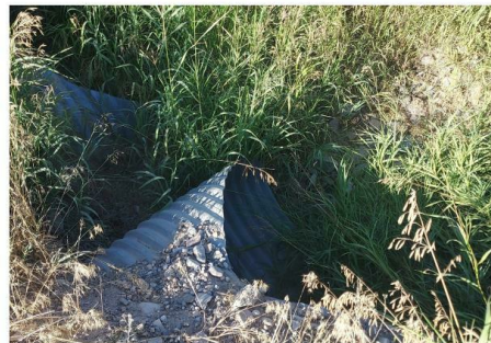
#35. VIEW OF SW CULVERTS
