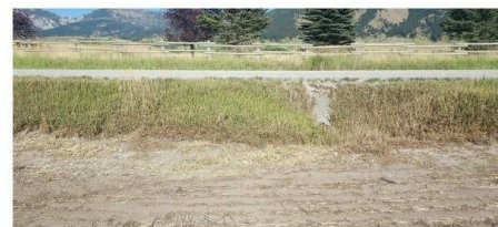
#51. VIEW OF EAST SE CULVERT
